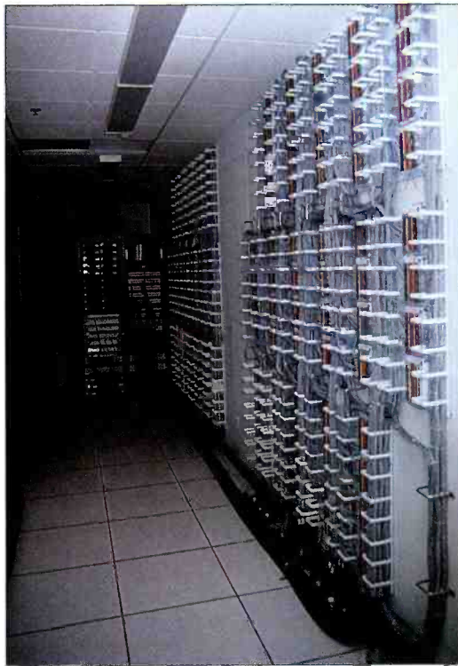
Racks are interconnected with 26-pair cable to wiring blocks mounted on the wall behind each technical area. Computer flooring makes wiring changes a snap.
